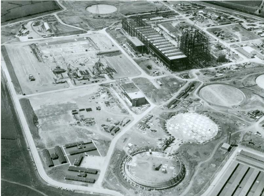
Plate 18: West Burton Power Station during construction in 1963, facing north
