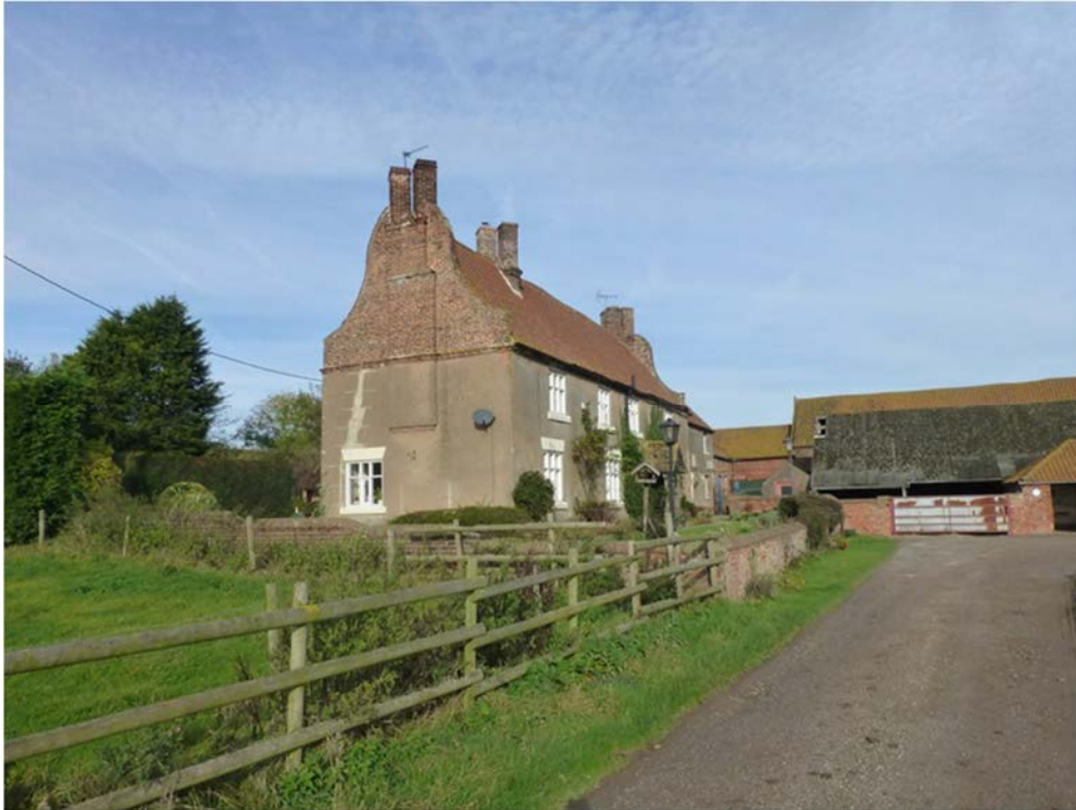
Plate 8: Grade II Listed Bole Manor House and attached outbuildings, looking north-west
