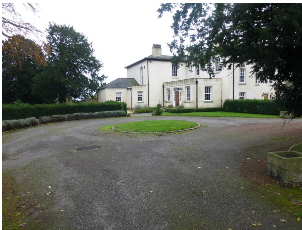
Plate 6: Grade II listed The Grove, Saundby. looking east
