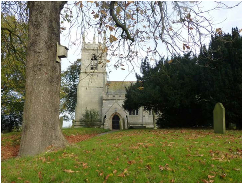
Plate 10: Grade II Church of St Martin, Bole, facing south
